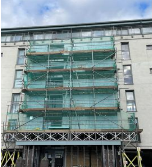
Picture showing Vincent House progress with completed insulation on upper level.
