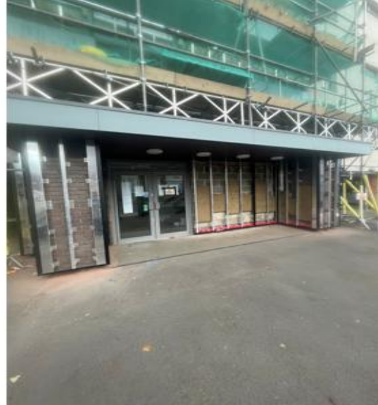
Picture showing fire barrier and insulation to ground floor begin install
