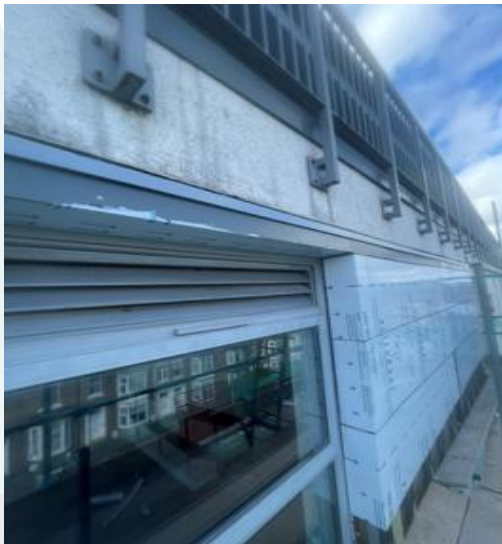
Picture showing top level panels installed and sill to head complete
